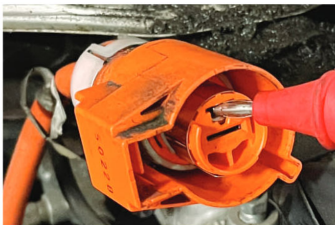
Testing one of the two DC cables with an insulation test meter.
