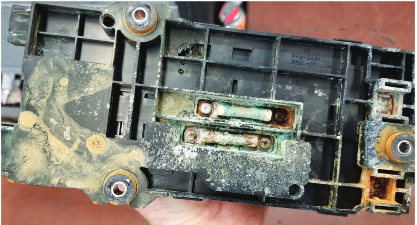
This Highlander Hybrid system main relay didn't survive an over-zealous seat shampoo at a detail shop. It drove in but couldn't drive out. Both the Highlanders and the RX400hs have the system main relay in a low spot under the rear seat. A P0AA6 can be caused by water leaks at the rear hatch, spilled soda, or anything that wets the rear seat.
